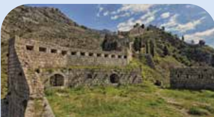
WALL OF KOTOR
